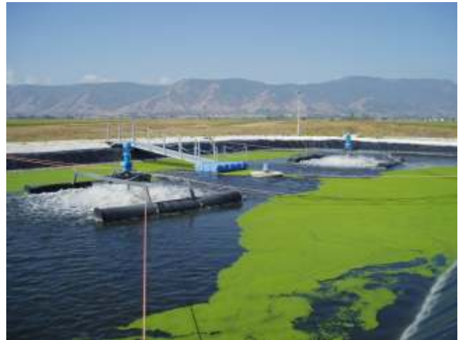
Waste water treatment plant
